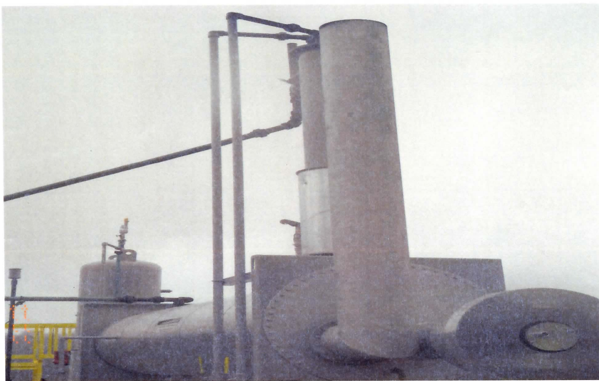
6. Still Vent & Reboiler Stack 40MMscf/day dehydrator – LMM Springhill CS – 11/10/2015
