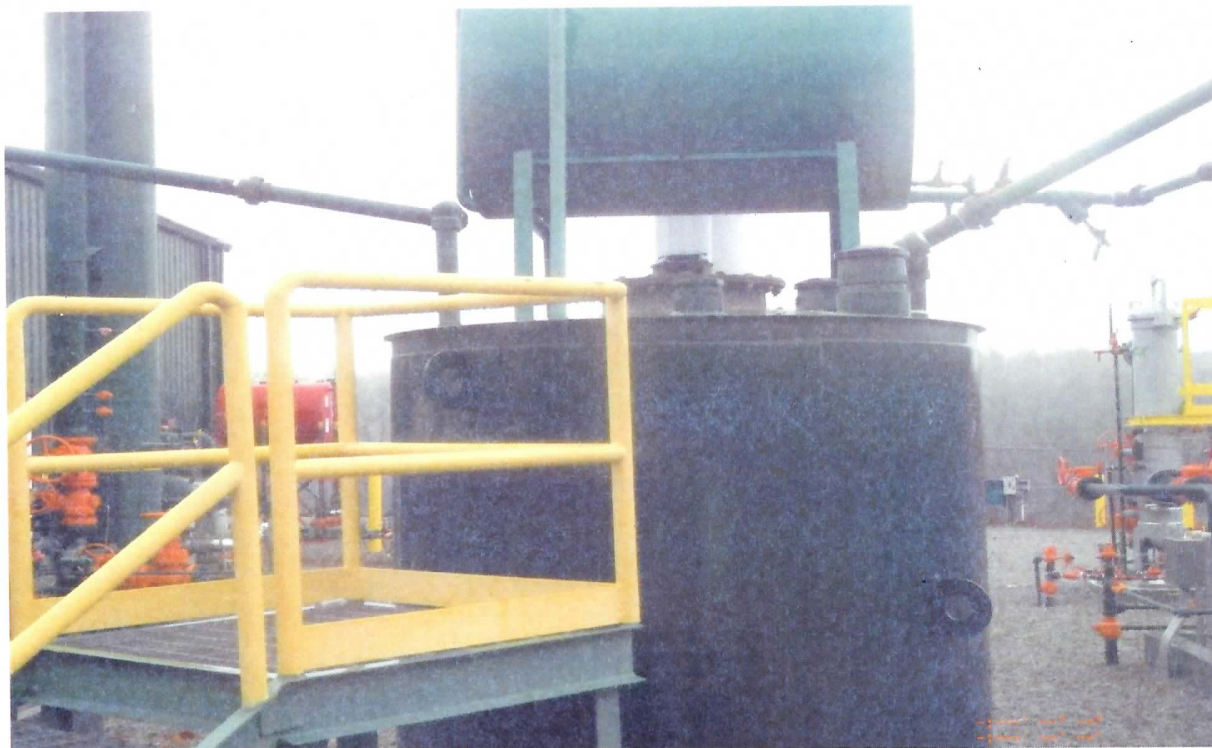
5. Produced Water Tank between Two Glycol Dehydrators – LMM Springhill CS – 11/10/2015
